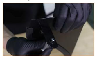
04. Locate the small bracket in your kit, and install a mounting peg to the slotted hole on the bracket. Leave it slightly loose to allow for adjustment. (1x long 4mm Allen bolt, 1x lock washer, 1x large flat washer)
